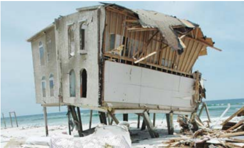
Dennis strikes Navarre Beach, FL, Photos by: Leif Skoogfors, FEMA
